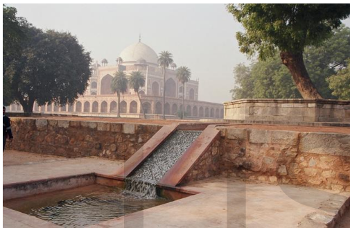
Figure 20: Water channel and pool after restoration
