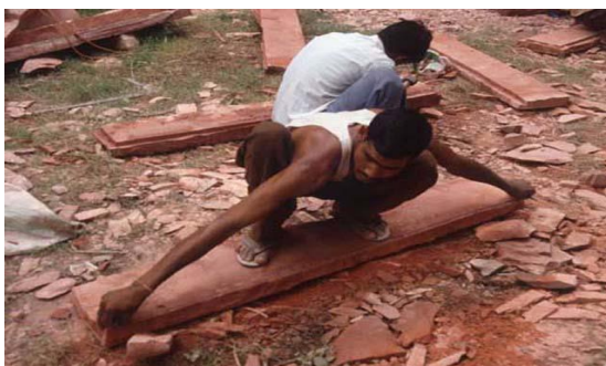
Figure 21: Edging stone restoration
