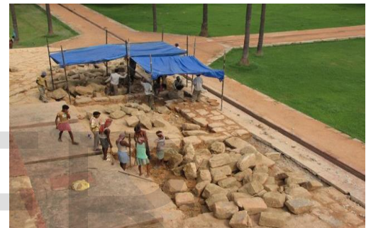
Figure 22 : Restoration of plinth which acts as an interface between the tomb and the garden.
