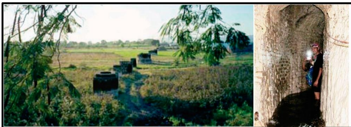
Figure 16: Series of air shafts and Underground channels
